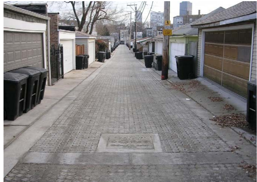
Examples of green multi-use alleys and permeable pavings Photos: NACTO
