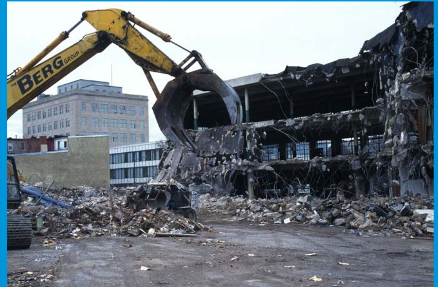
Demolition of the Chesapeake Cadillac building Photo: John Dean
